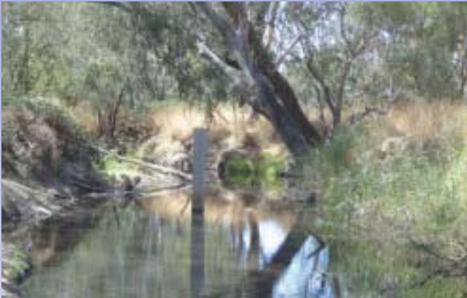
During works inspection, with driven piles mid stream.
