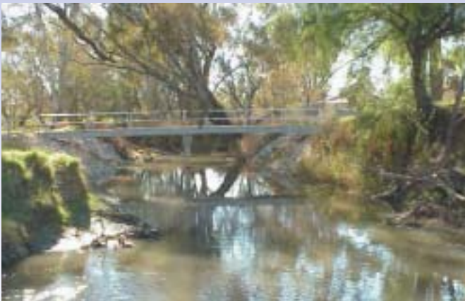
Completed pedestrian bridge constructed in accordance with a permit for works on waterways.
