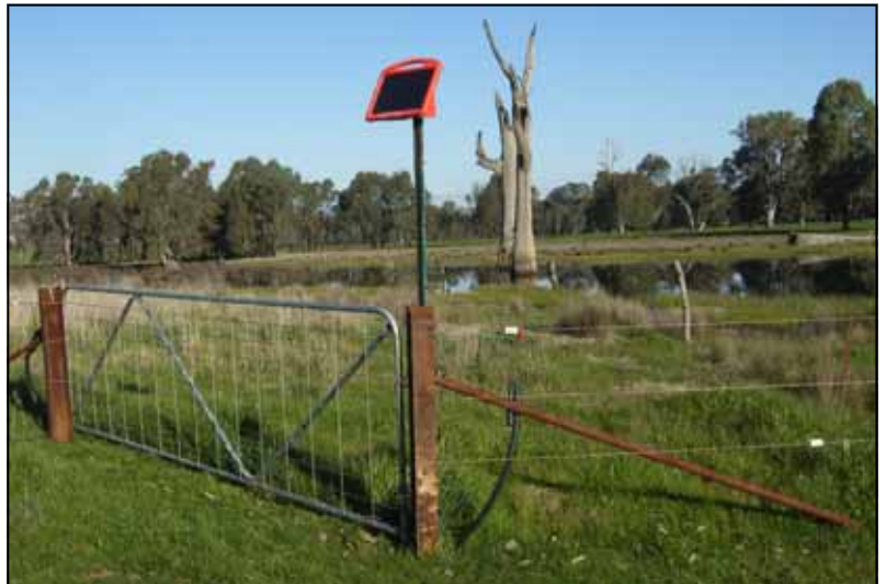
Photo 1: The fence protecting this wetland has been designed to be flood resistant. Very strong end assemblies of railway iron support a minimal framework of three electrified plain wires powered by a stand-alone solar-powered energizer.
