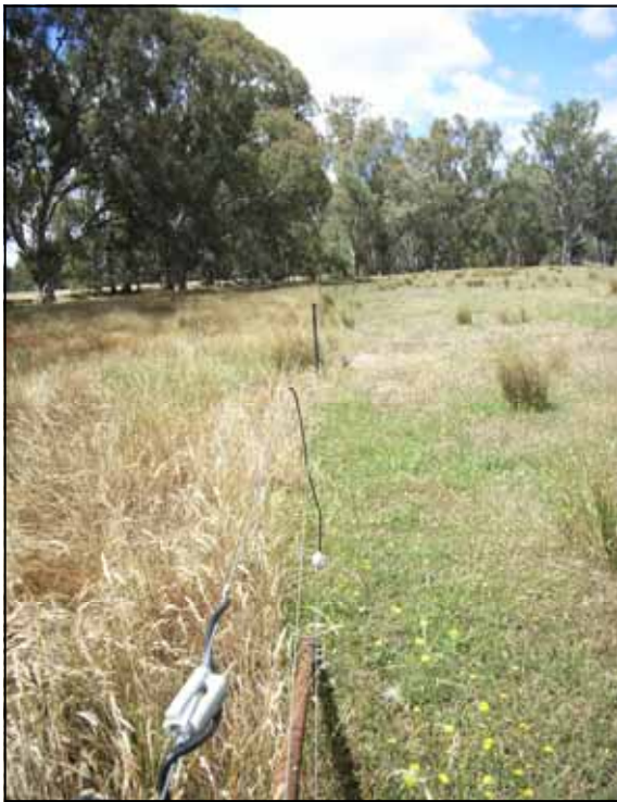
Photo 11: This fence has been positioned well away from overhanging trees. This has two benefits; firstly damage from falling limbs is greatly reduced, and secondly by moving the fence further back from the creek straighter runs of fence are possible. This reduces the number of expensive corner assemblies that are required.
