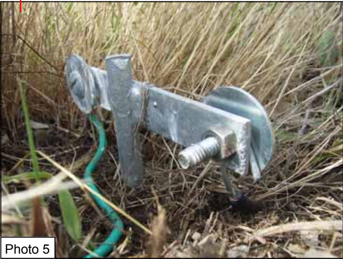
Photos 3-6: Wires are not run through the star pickets themselves but are attached to the pickets on the downstream side of expected flood flows (photos 3 & 4 above). The wire will be more likely to release from the picket if it is struck by debris, rather than pulling the star picket out. Photo 5 (bottom left) shows a close-up of a galvanized earth spike. Proper earthing of electric fencing is vital to ensure maximum performance and a minimum of three, inter-connected 2m long earth spikes should be fitted. Photo 6 (bottom right) shows how flexible the fence is where droppers are used - this allows debris to flow through the fence with less likelihood of it snagging the wires. This type of fence is ideal for situations where flood flow direction is unpredictable.
